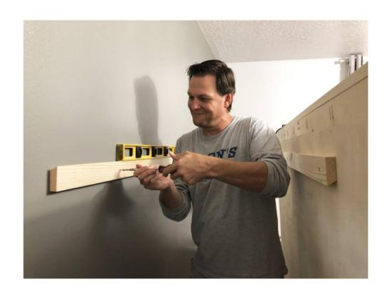
To ensure that the headboard is secure, we used a French cleat to attach it to the wall. Cut a 2x6 in half at an angle. Screw one to the wall and one to the back of the headboard. Then lift the headboard up and set it down onto the cleat on the wall.
